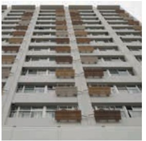
Air conditioner coverings
