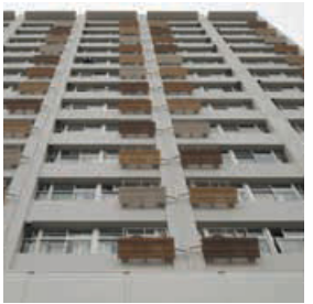
Air conditioner coverings
